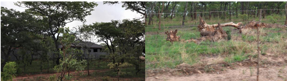
Picture left: Construction happening in the forest
